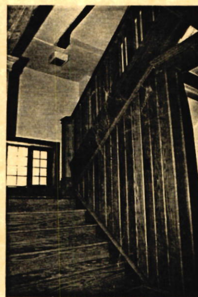
After: The stairway's oak woodwork has been uncovered and refinished. The window has been replaced with the original type of sixteen-paned window consistent with the other windows of the house.
